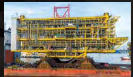
Central Processing Facility Fixed Platform Topside
