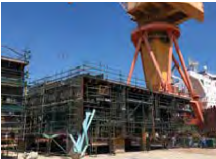
Johan Castberg FPSO structural blocks
