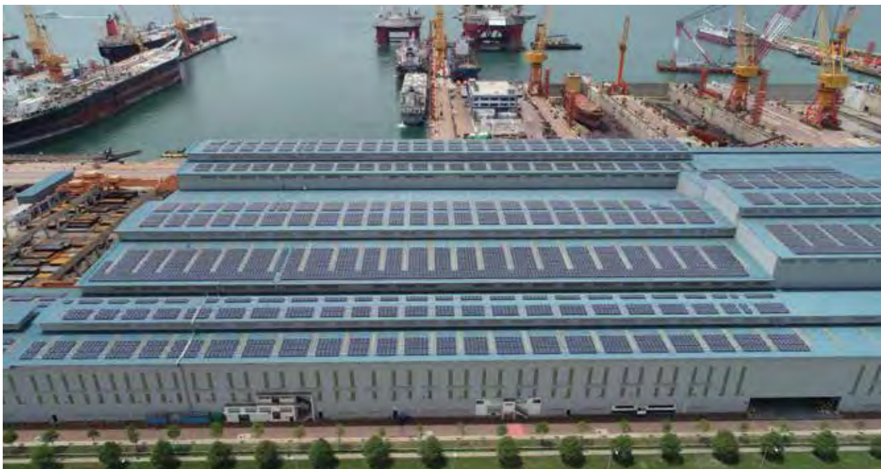
Sembcorp Marine has collaborated with one of Singapore's largest energy providers to install a 4.5 megawatt-peak solar farm and a digital energy saving system at Tuas Boulevard Yard
