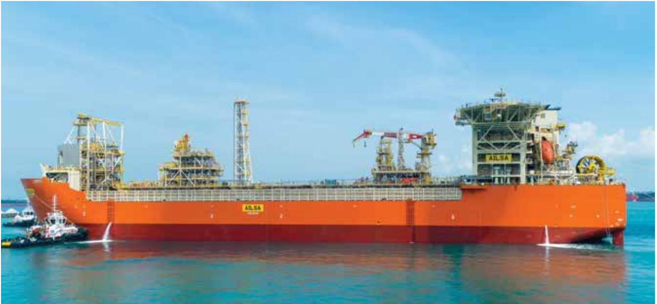
FSO Ailsa was delivered to MODEC in 2Q2018 for deployment at the TOTAL-operated Culzean field in the UK North Sea
