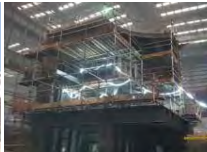
Karish FPSO hull fabrication
